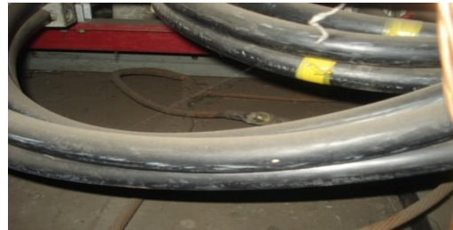
Fig.21 CPT's en tablero TPP-TR-4
