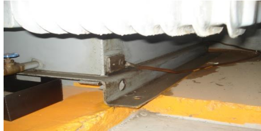
Fig.20 Conector a tierra del TR-3
