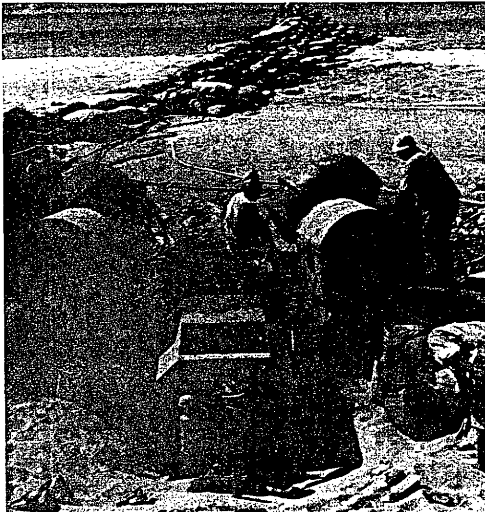
The new method saves time, cost and labor, yet uses very little equipment. Here two small concrete mixers and a pump fill the Bolsacreto forms with concrete made from local sand and gravel.
