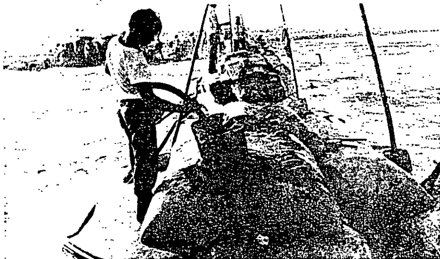
Filling a 3.5-ton Bolsacreto at Port Sanchez Magallanes through the reinforced protuberance.
