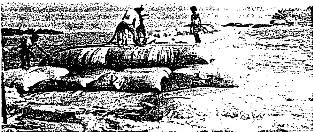
Bolsacreto breakwater under construction requires little labor. Several breakwaters have survived hurricanes with no damage.
