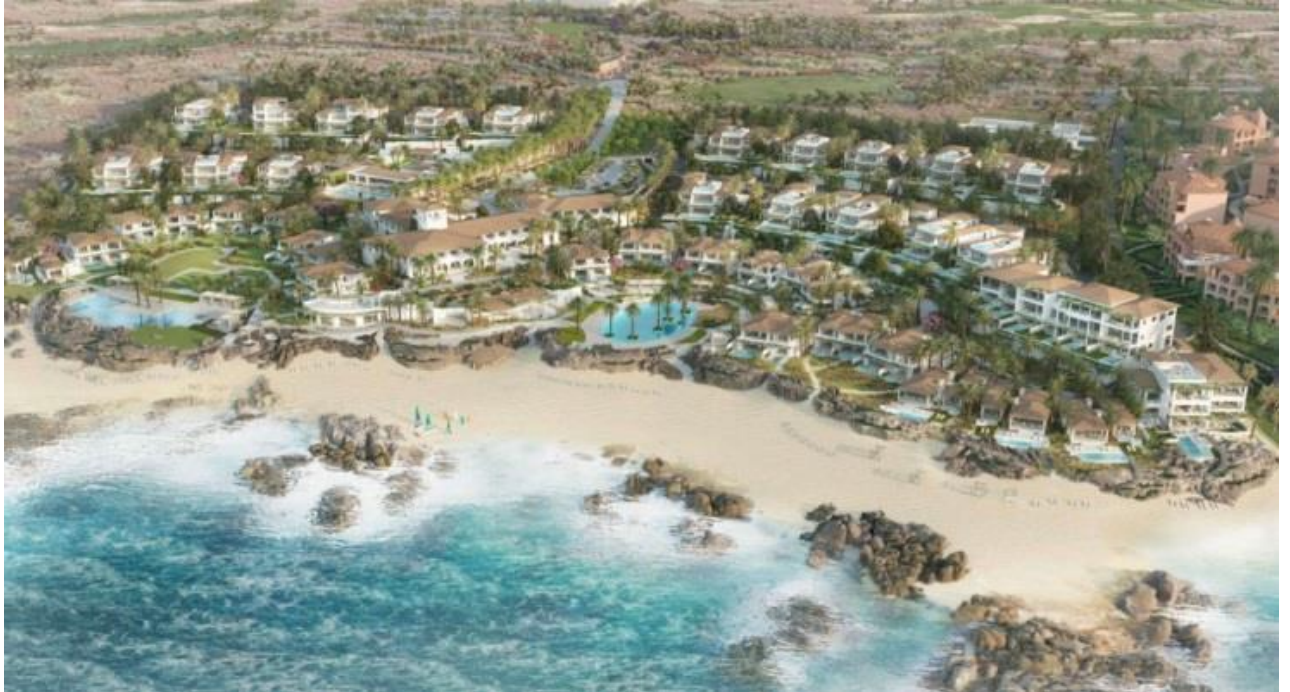
Figura 2. Complejo Four Seasons, Cabo del Sol
