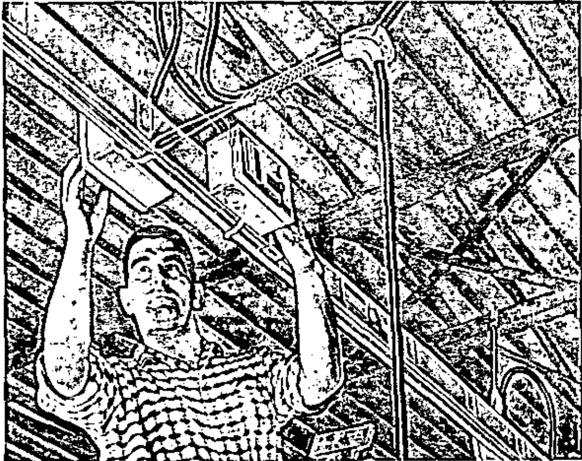
Figure 9.19 An Installation View of Medium-Current Plug-in Busway Showing Individual Short-Circuit-Protected Power Take-Off Cables
