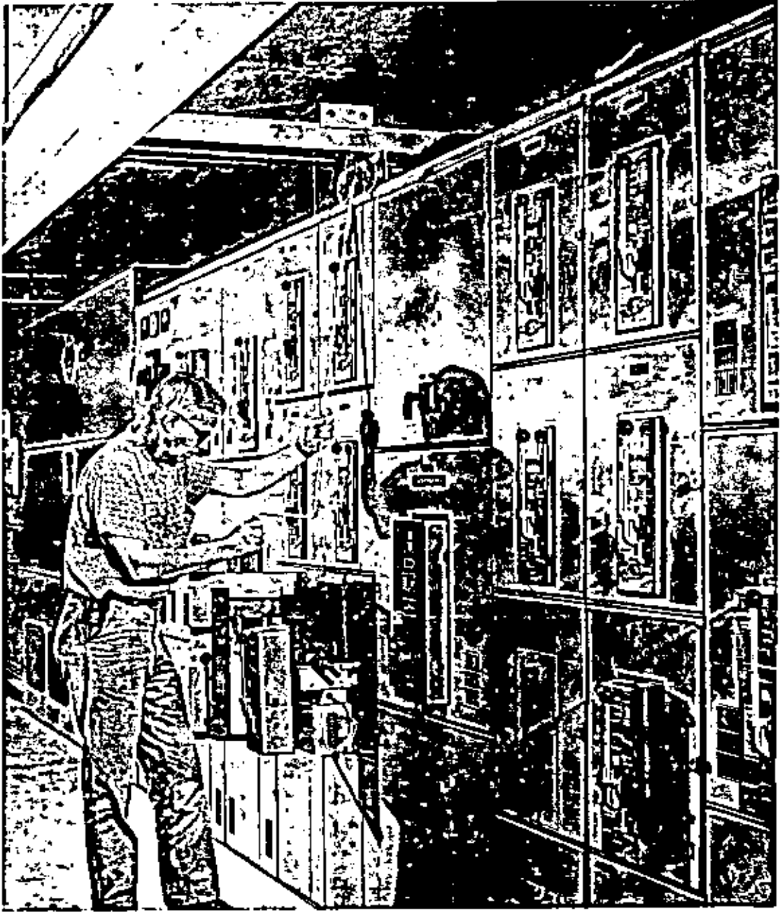
Figure 7.2 Installation of low-voltage draw-out switchgear
