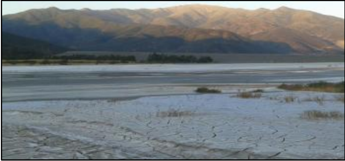
Figura 4. 11. Depósito de jales en pasta de la unidad Alhué, Chile. Fuente: Sustainable Management of Thickened Tailings in Chile and Peru: A Review of Practical Experience and Socio-Environmental Acceptance (Cacciuttolo & Marinovic, 2022).
