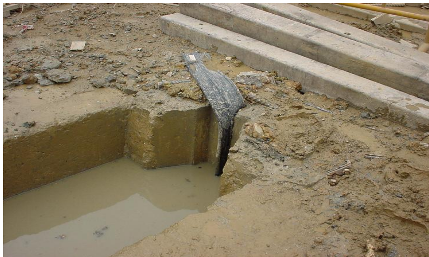
Junta Impermeable CWS.
