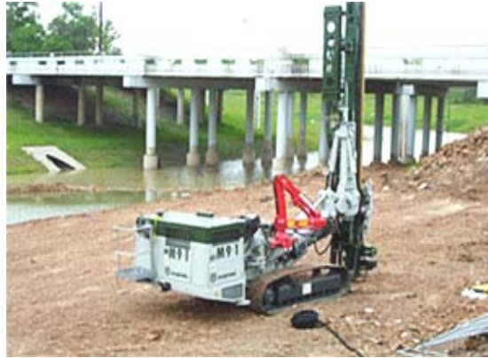
Fig. 1.15 Empleo de Jet Grouting.
