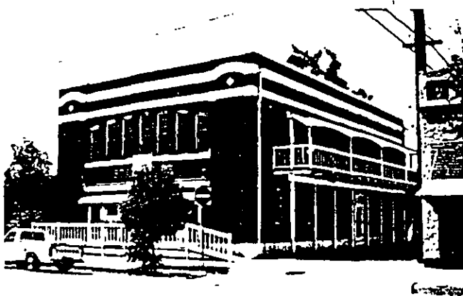
Figure 1. Southeast view of firehouse.
