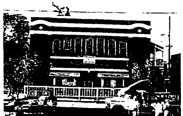
FIG. 1. South Elevation of Gilroy Firehouse
