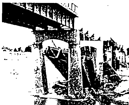
Photo 2-2 Falling off of Girders due to 1948 Fukui Earthquake
