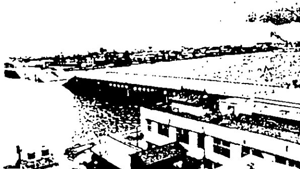
Photo 1-3 Damage of Showa Bridge by the Niigata Earthquake of 1964
