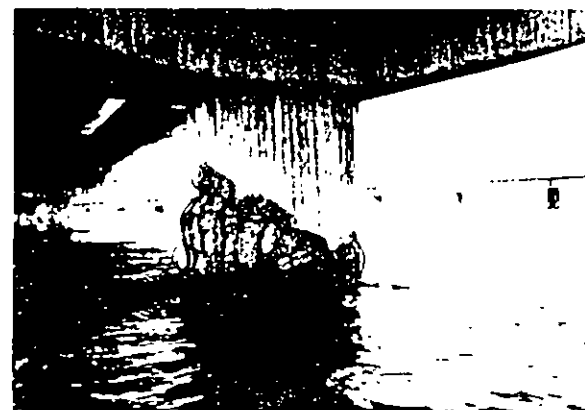
Photo 1-7 Damage to Reinforced Concrete Piers of Shizunai Bridge by the Urakawa-oki Earthquake of 1982
