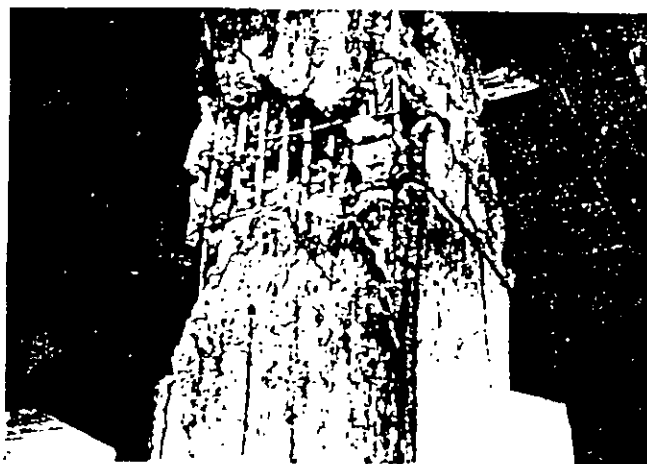
Photo 2-4 Earthquake Damage to the Column of Railway Elevated Bridge by 1978 Miyagi-ken-oki Earthquake
