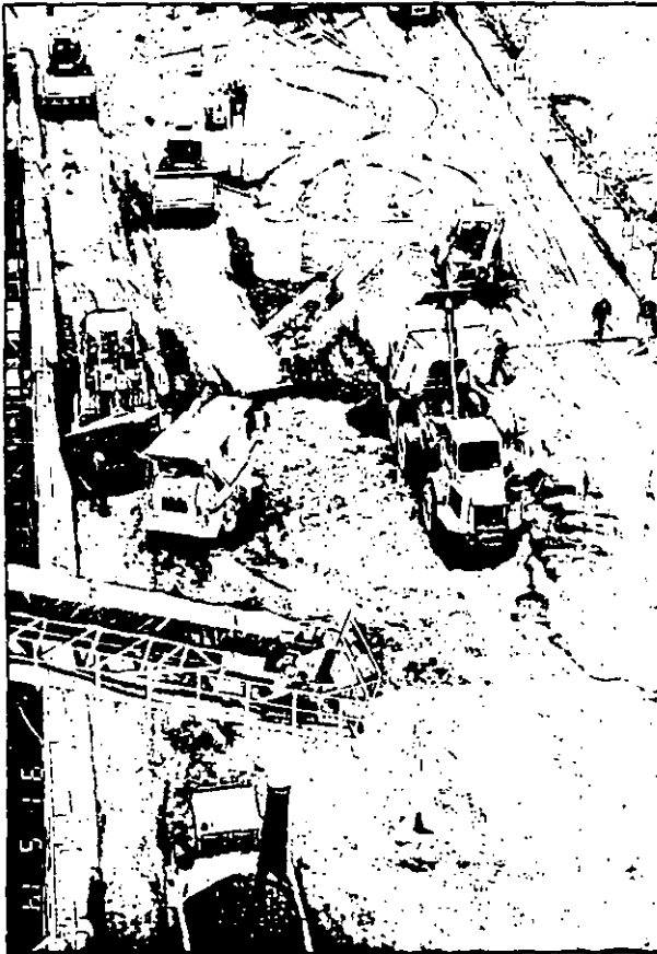
Typical RCC placement operation in May 1991.
