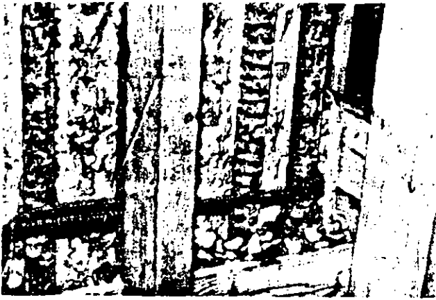
Fig. 11—After damaged concrete has been removed, coarse aggregate is placed as timber forms are erected
