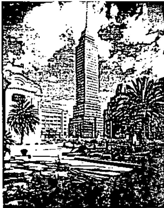
Latin American Tower, Mexico City, Mexico—example of steel moment-resistant frame (Courtesy W. E. Edwards, Bethlehem Steel Co.)
