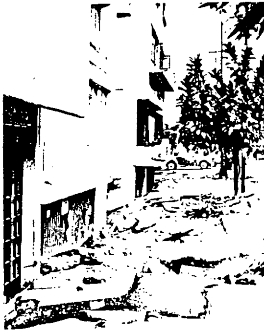
Figure 4 - Settlement of Building Ib.
