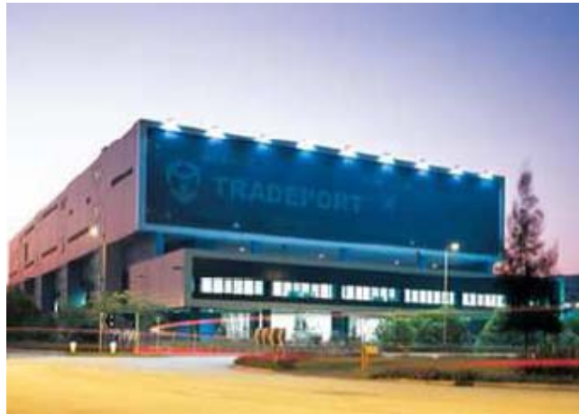
Figura 5-34 Tradeport Logistics Centre Fuente: Airport Authority Hong Kong
