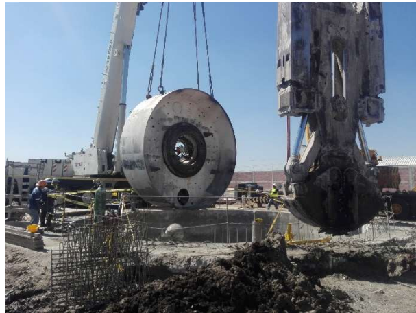
Figura II.53. Almeja guiada, [Cortesía ICA, Ing. Victor Yeo]
