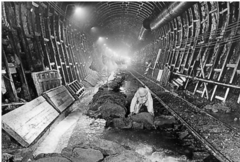
Figura 1.43. Túnel Emisor Central. Ref. [77].
