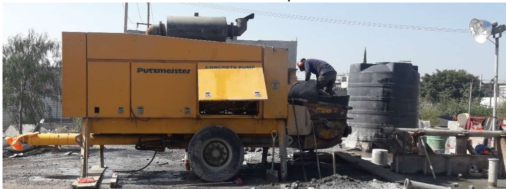
Figura II.60. Bomba de concreto Putzmeister BSA 14000, [Propia]
