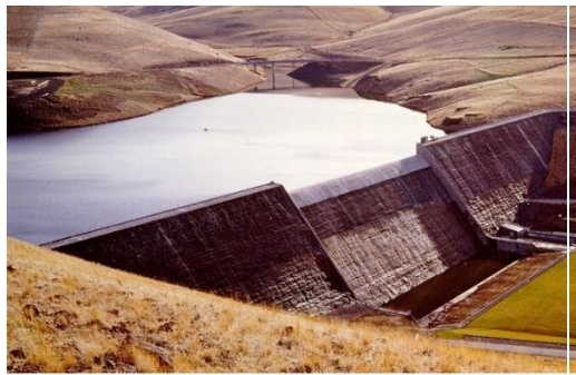
FIG. 4.2 PRESA WILLOW CREEK
