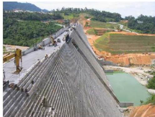
pre-cast block forms for 0.6m d/s steps for SLM in 3m lifts
