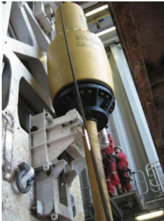
Figura 30.- Flexible Joint Installation
