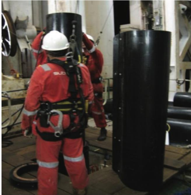
Figura 29.- VIV Fairing Installation
