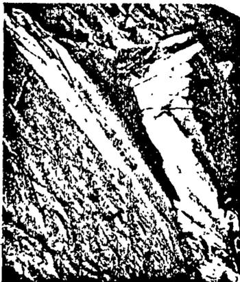
Figure 2: Wedge failure in a hard rock slope involving sliding along the line of intersection of two discontinuity planes.
