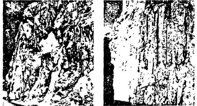
Figure 3: Damage to a rock face by excessively heavy blasting giving rise to rockfall instability.
