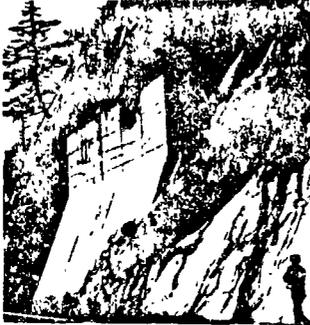
Figure 9: Concrete buttress to support rock.
