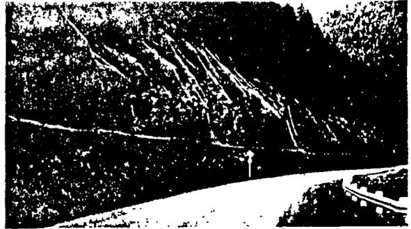
Figure 11: Wire mesh draped over a blocky rock slope.
