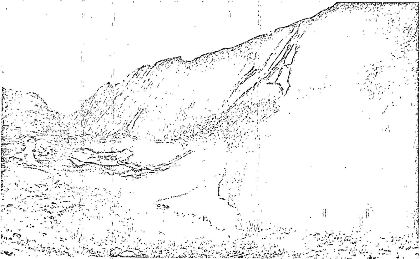
Fig. 45. Downstream view of landslide dam created by multiple HE detonations (total yield 1.2 kt) by Soviet engineers on Vakhsh River Reprinted from *Engineering News-Record*, May 30, 1968, copyright McGraw-Hill, Inc. All rights reserved.
