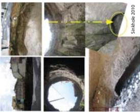
The subsidence phenomena occurred in February 2007 and May 2010 (respectively). In appearance both sinkholes were related with a rupture in the western drainage main collector, supposedly a rupture and/or an explosion caused by gas accumulation gave origin to the sinkholes.
