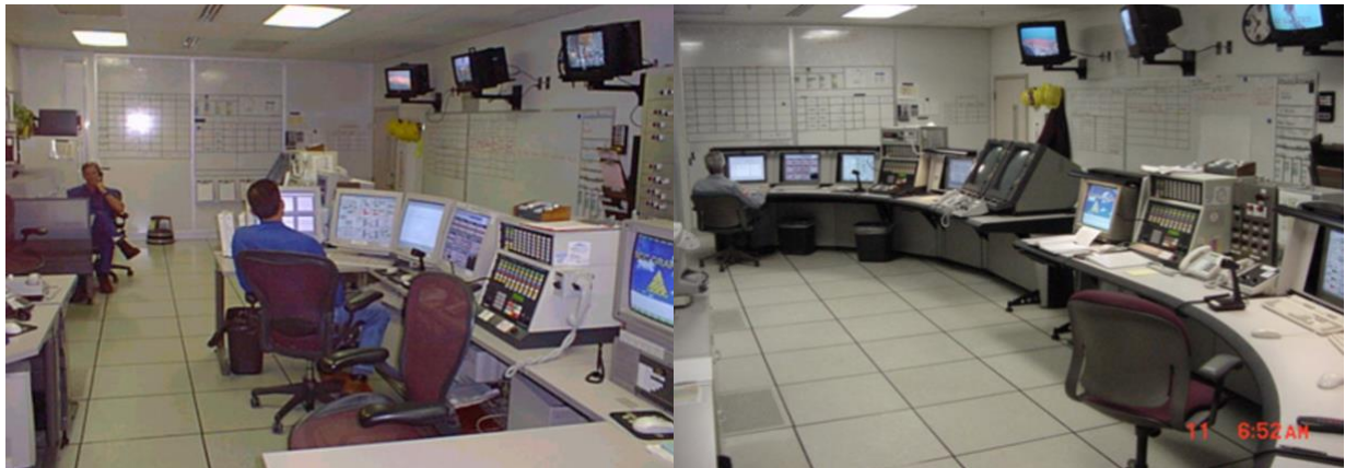
Figure 11. Control room design with inadequate (left) and adequate (right) workspace from an ergonomic perspective. (IOGP, 2011)
