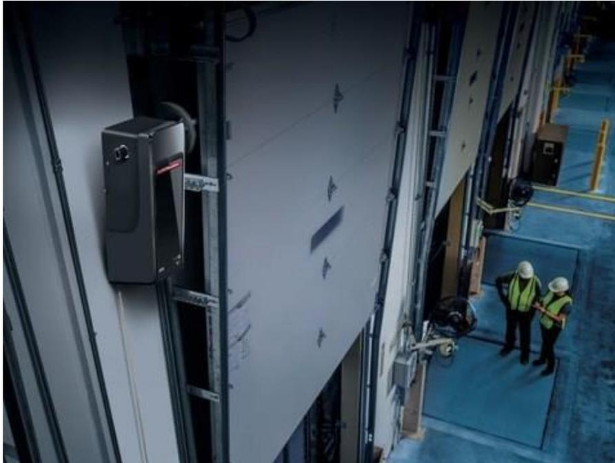
Figura 2. Abridor de puerta comercial DDO8900W controlado controlado por cadenas [Fotografía], por Cision, 2019 (Tomado de <https://www.prnewswire.com/news-releases/liftmaster-introduces-dock-door-operator-with-cloud-based-access-and-dock-management-capabilities-300897113.html>)
