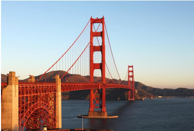
Figura 1.4 Puente Golden State, U.S.A.
