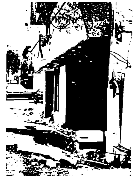
Fig. III-4.3: Earthquake induced tilt and settlement of a building on a partially compensated foundation
