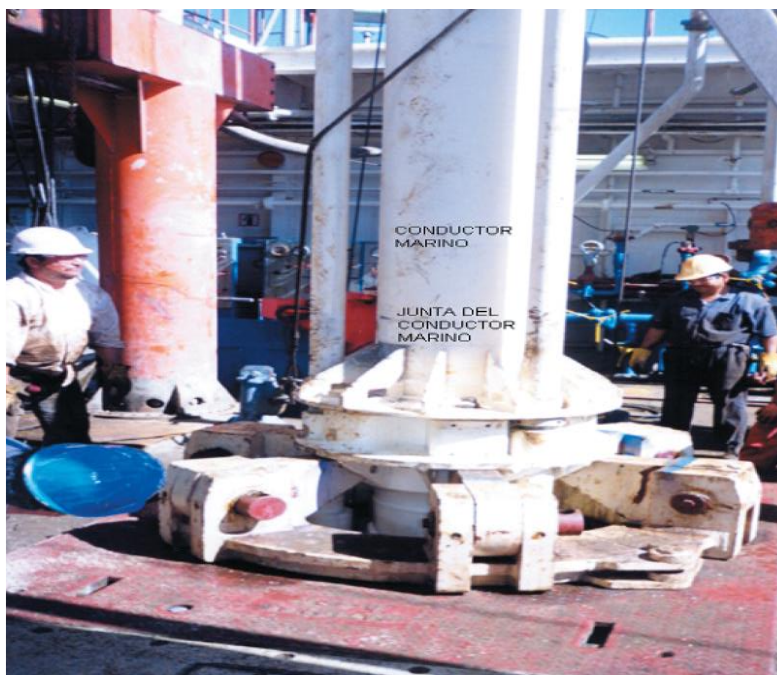
FIGURA 17. CONDUCTOR MARINO (RISER)
