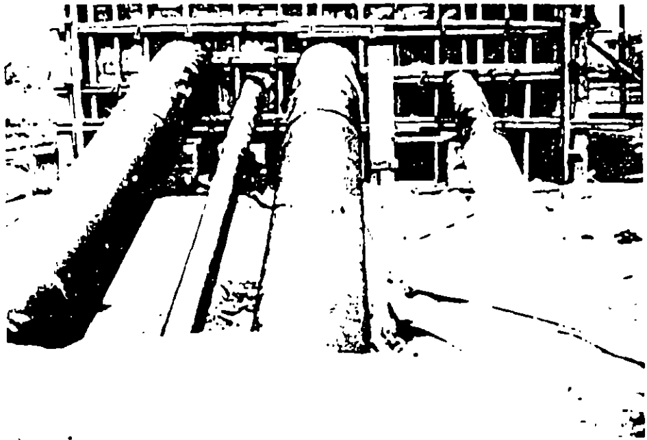
Figure 5.44 Primary leachate collection sump side wall riser pipes leading from sump into collection and monitoring shed.
