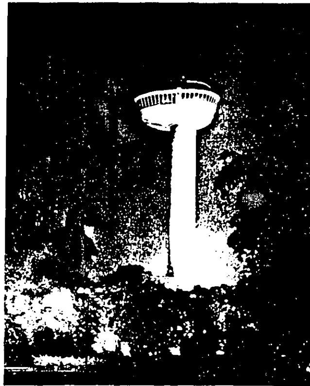
Fig. 44. High lighthouse towers, often with a restaurant at the top, are very rewarding subjects for a floodlighting system. The floodlights, however, must not impede the view from the restaurant. A steep angled arrangement of narrow beam light sources located at the foot of the building lights up the tower and makes it visible from far away. Because of the glaring light, the pattern of brilliance on the tower changes markedly with height effect. Carefully bringing out the rounded form of the building.
