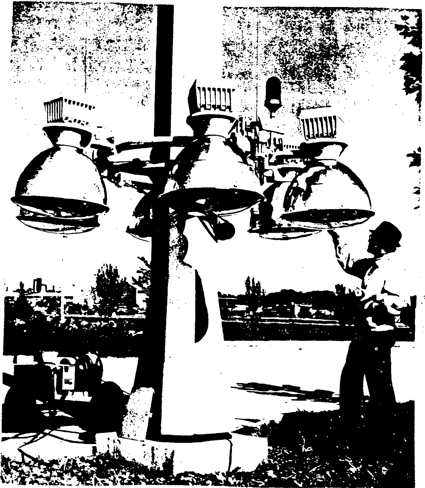
Fig. 6-15. High-wattage, high-mounted, area-lighting luminaires.
