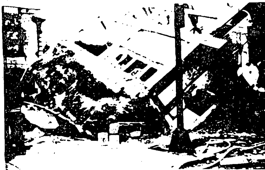
Figure 12 - View of collapsed Building V.
