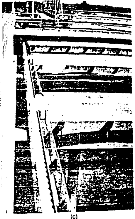
Figure Effluent Weir, Notches, Launder, and Outlet Channel in Rectangular and Circular Clarifiers. (a) V notches and suspended effluent launder in circular clarifier. (b) Effluent launders discharging into an outlet channel. (c) Effluent notches, launders, and outlet channel in a rectangular clarifier.
