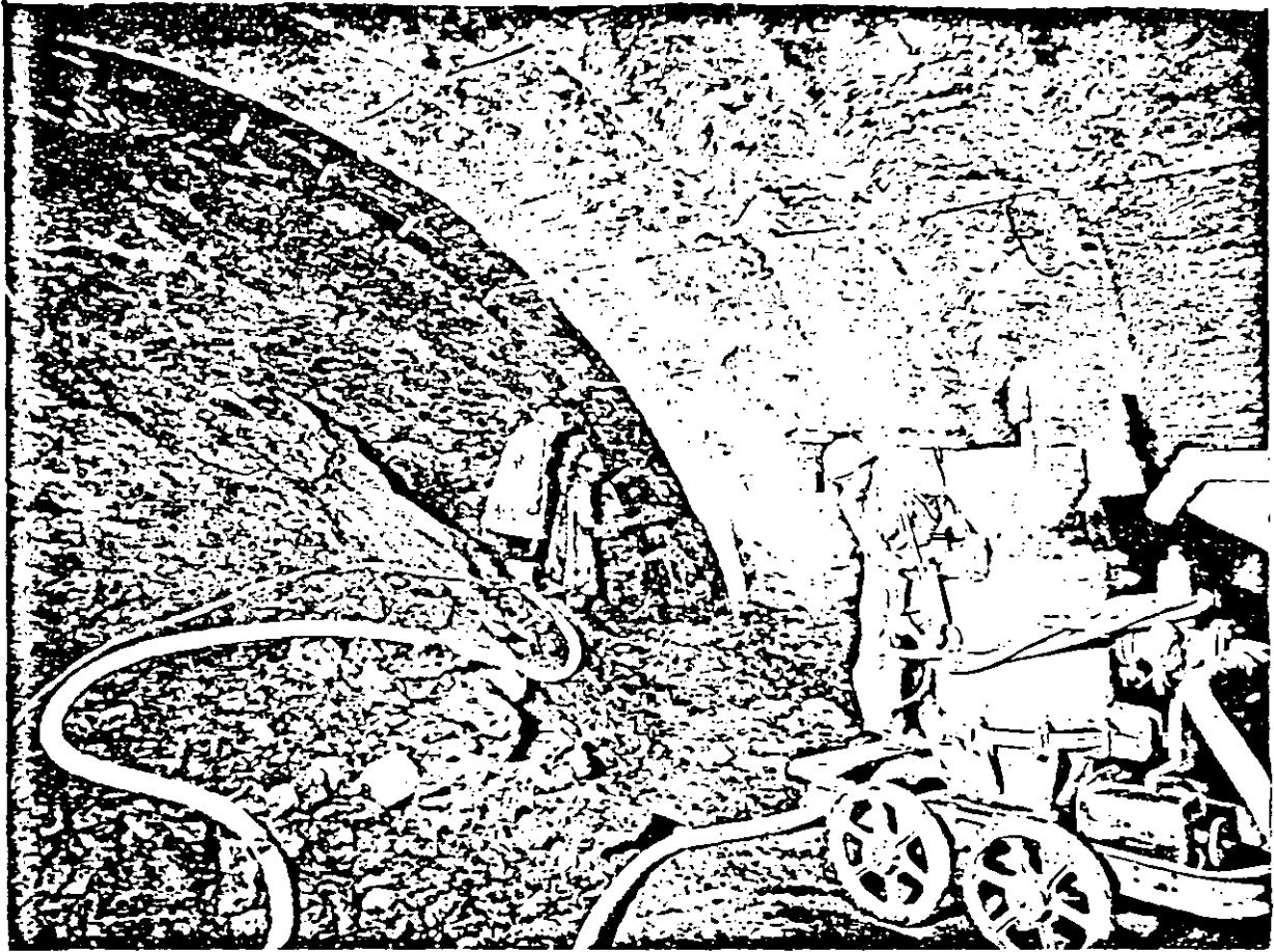
Fig. 19. Super-highway tunnel in Italy south of Firenze. Forming the auxiliary lining of the upper part of the tunnel with shotcrete reinforced by steel netting and steel arches. Contractors: Impresit G. Lodigiani, Milan
