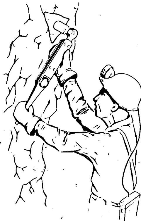
Fig. 5 Tensioning of an expansion shell anchored rockbolt using a torque wrench.
