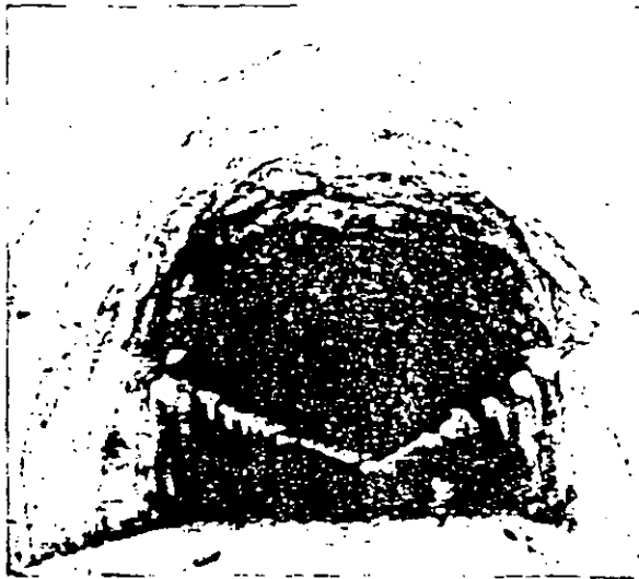
Fig. 30. Permanent shotcrete lining of a super-highway tunnel in Venezuela, following the irregularities of the rock
