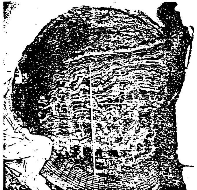
Fig. 29. Test gallery face (Schwaikheim) showing typical appearance of marly clay. Note the Shotcrete cover already placed in the foreground
