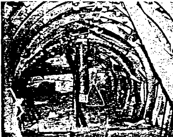
Fig. 3. Steel-supported tunnel which failed when reaching a zone of kaolinised gneiss under an overburden of 250m: water inflow 35lit/s
