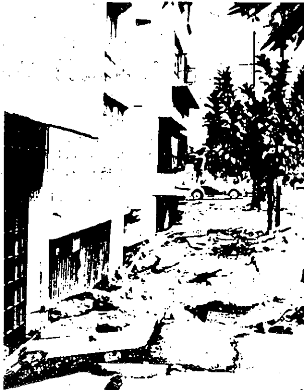
Figure 4 - Settlement of Building Ib.
