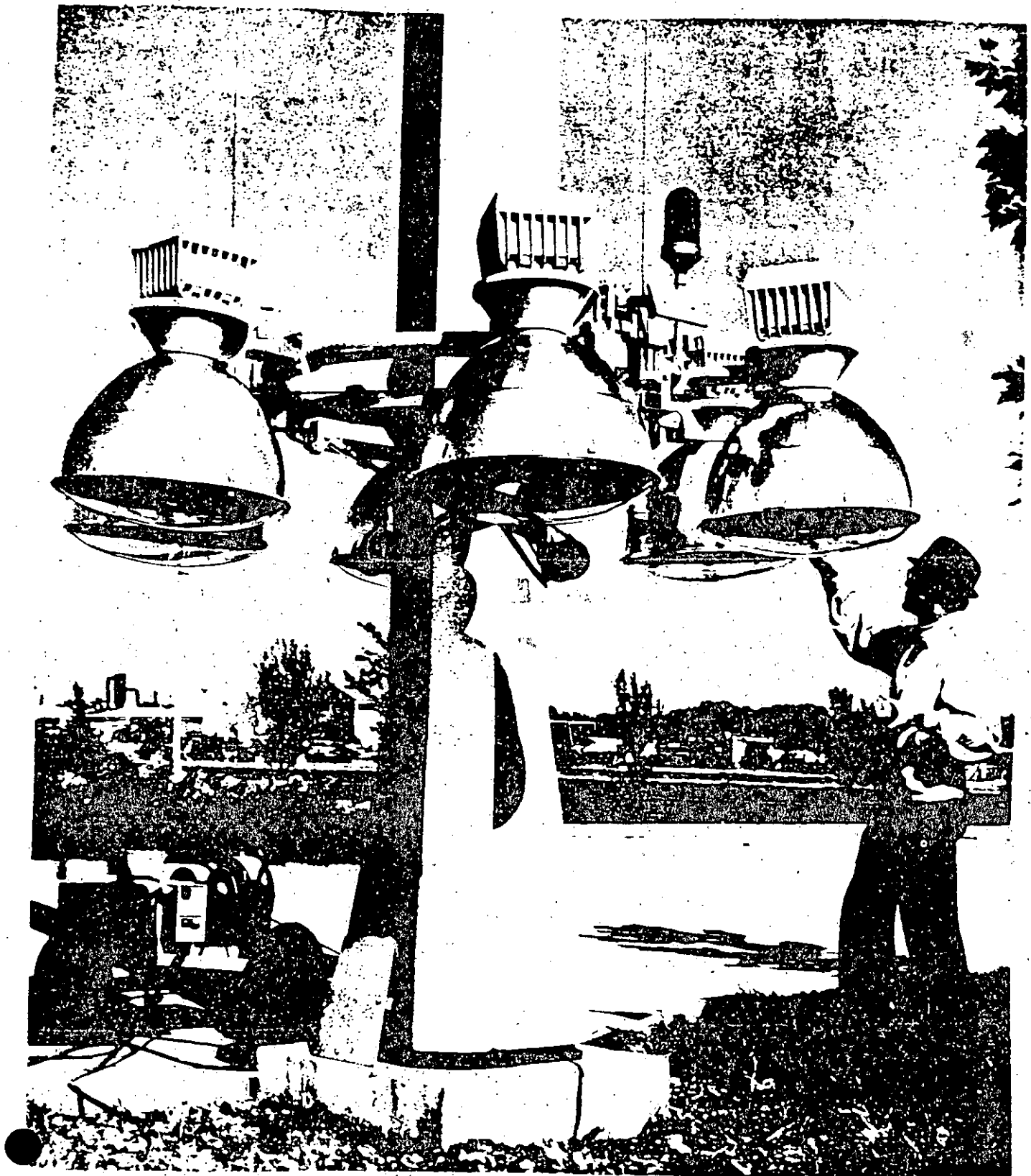
Fig. 6-15. High-wattage, high-mounted, area-lighting luminaires.
