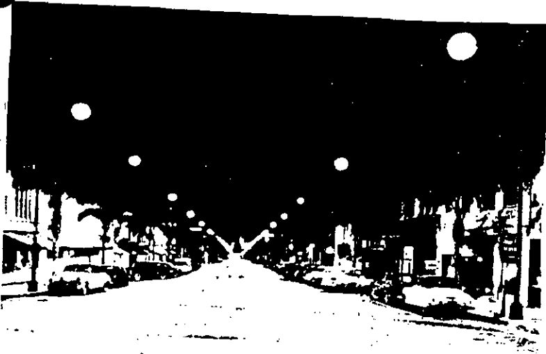
Fig. 7-14. Luminance pattern - opposite arrangement.
