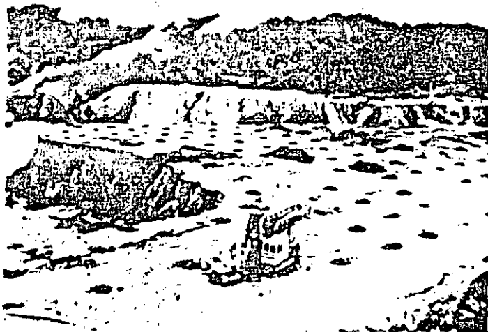
Preparation for a large production blast in an open pit mine. The dark coloured mounds are piles of chippings which have been air-flushed from the large diameter holes drilled to accommodate the explosive.
