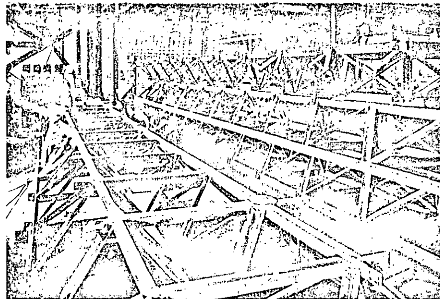
Welding of space trusses—Upjohn Company Office Building Courtesy Whitehead and Kales Company, Detroit.
