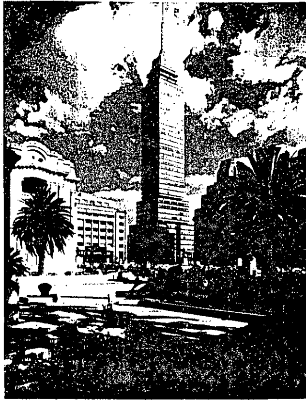
Latino Americana Tower, Mexico City, Mexico—example of steel moment-resistant frame (Courtesy: W. E. Edwards, Bethlehem Steel Co.)
