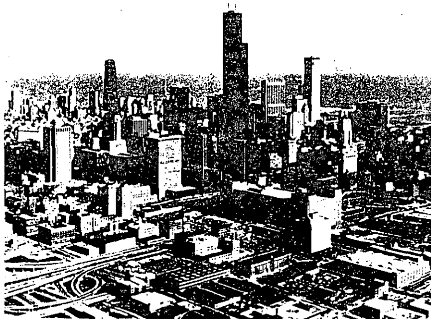
Examples in Chicago of three structural systems: John Hancock (braced tube), Sears Tower (bundled tube), and Standard Oil (tubular system) (Courtesy: Rita P. Krider & Engineering News Record)
