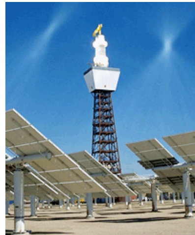
Torres de Receptor Central, Barstow, California.
