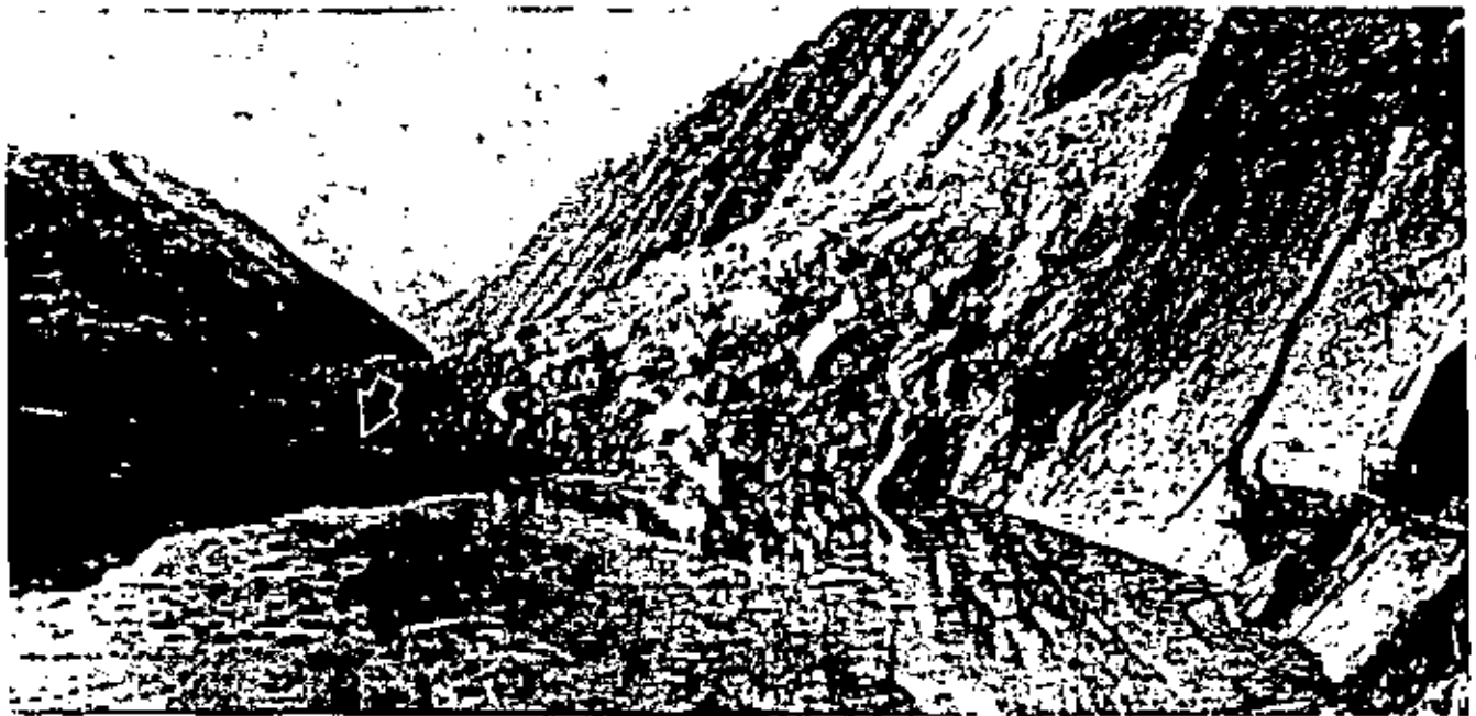
Fig. 47. Closeup of explosion-produced dam on the Vakhsh River. Reprinted from Engineering News-Record , May 30, 1968, copyright McGraw-Hill, Inc. (all rights reserved).
