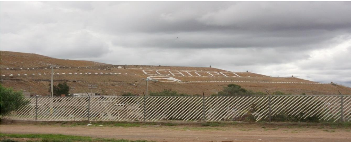
Figura 4.6 Relleno Sanitario Santa María Chiconautla, 2013
