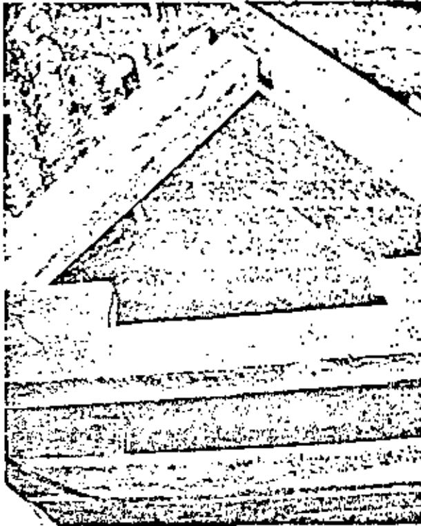
Figure 6 : "Cathedral" failure in the roof of a tunnel aligned parallel to the line of intersection of two well developed discontinuities.
