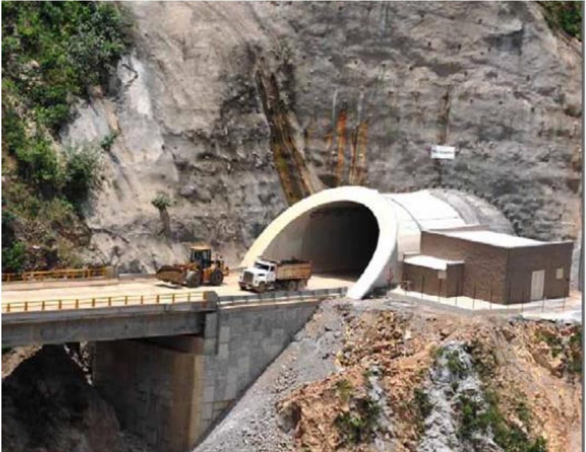
Fig. No. 161 Falso Túnel
