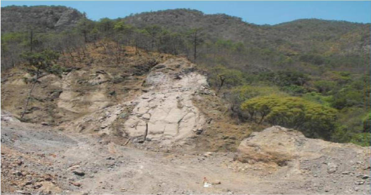
Fig. No. 40 Desmonte del portal Durango
