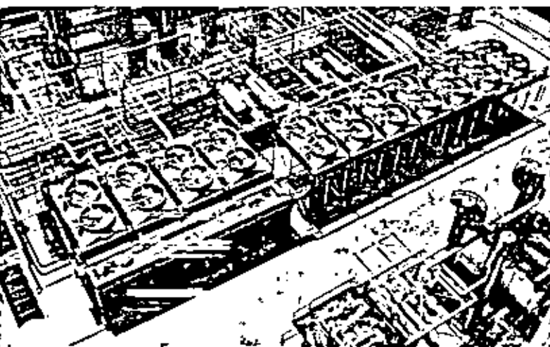
COMBIN-AIRE AND FIN-FAN units in a West Texas refinery dissipate over 250 million BTU'S per hour directly to air. Three similar COMBIN-AIRES have been installed within this refinery in addition to the unit shown above.
