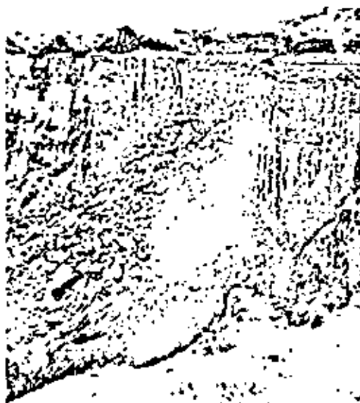
Upper slopes on the de Beer's diamond mine at Kimberley in South Africa. Failure of the vertically jointed dolerite is induced by progressive weathering of the underlying shales.
