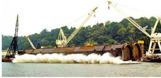
Figure 2.33 Side launching of a tube element (De Wit et al., 2012)
