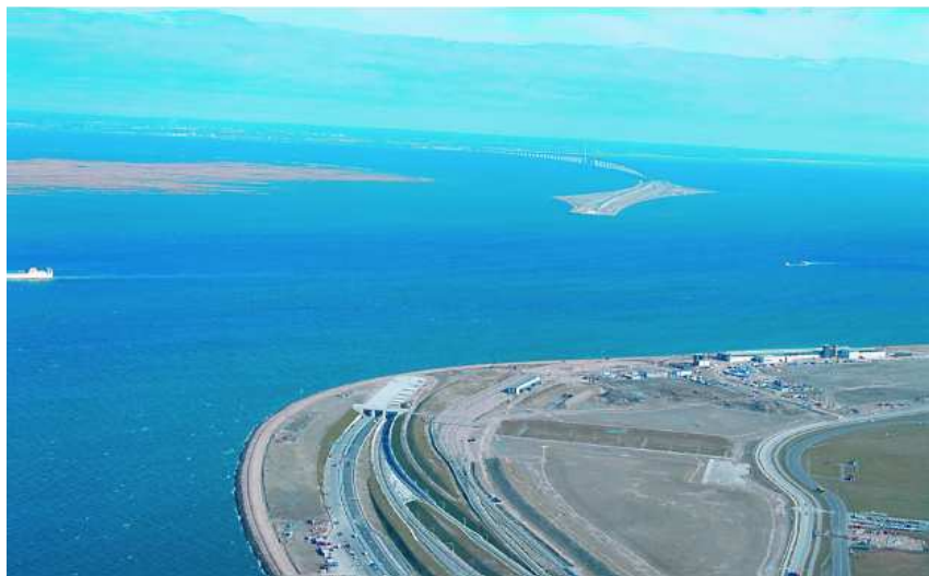
Figure 2.18 Aerial view of the Oresund Link (De Wit et al., 2012)
