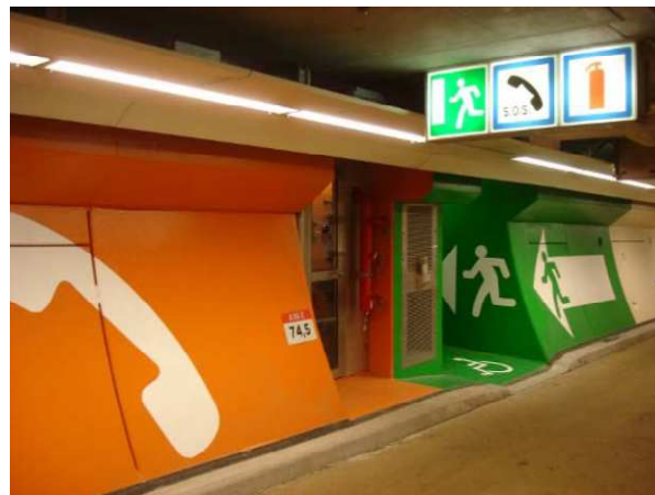
Figure 4.47 Configuration of the emergency station of the SFT of the Gulf of California (PIARC)
