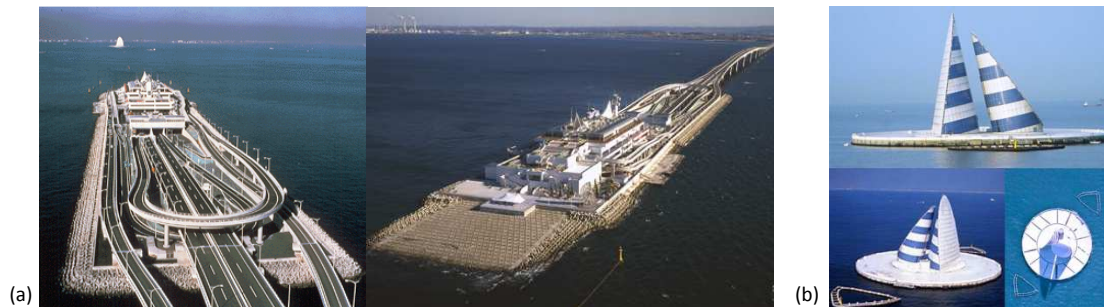
Figure 2.17 Artificial islands in the Tokyo Bay Aquiline: (a) The Kisarazu Island joins the subsea tunnel and the bridge; (b) The Kawasaki artificial Island works as ventilation towers. (dvice.com & findery.com)
