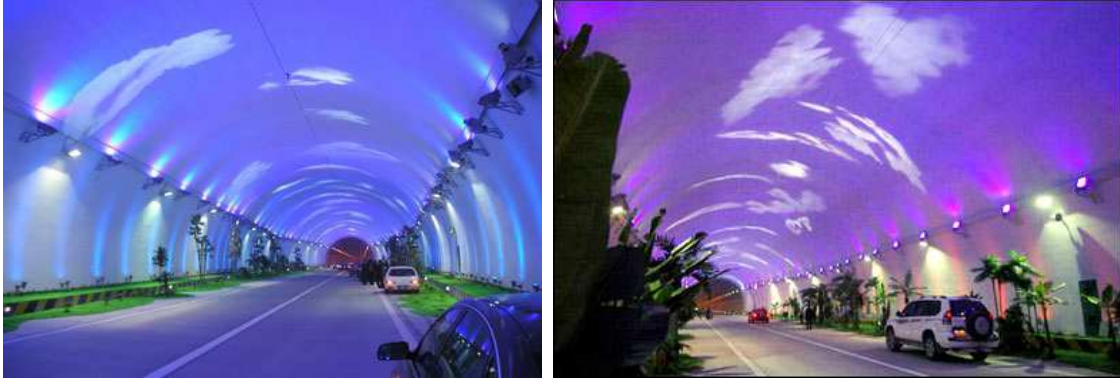
Figure 2.10 Interior design of the Zhongnanshan Tunnel (China.org.cn)
