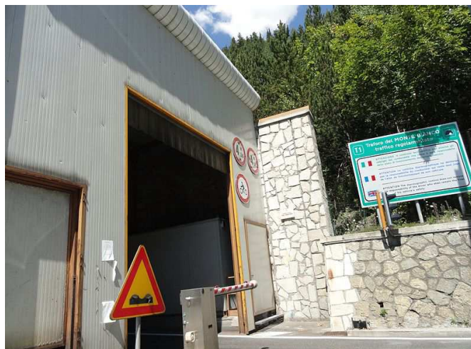
Figure 2.12 Thermographic inspection stations in Mont Blanc Tunnel (Kristoferb, 2011)
