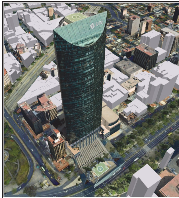
Figura 2.81: Torre Mayor, México, DF.
