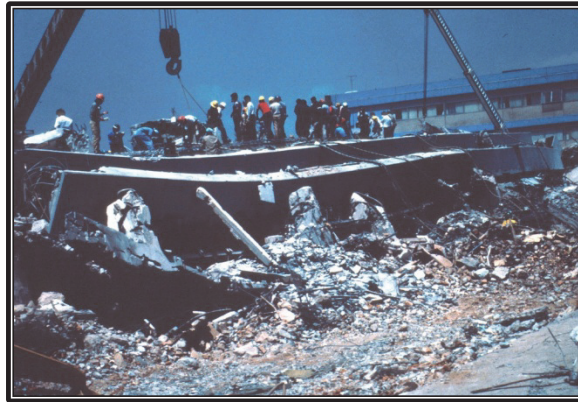
Figura 3.13: Colapso del Hospital General de México, México, DF. (Ref. V)
