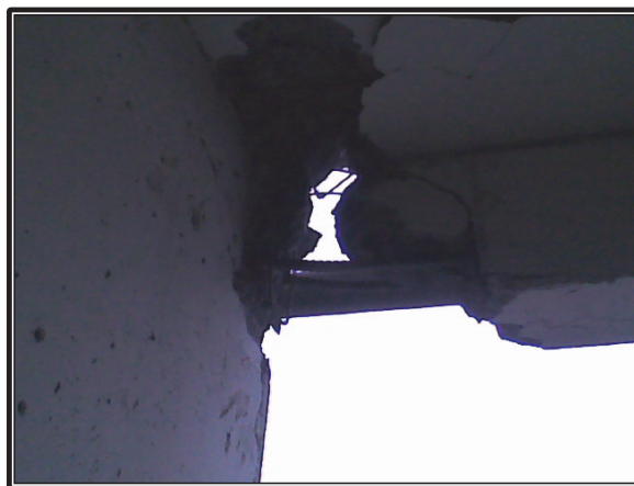
Figura 3.54: Edificio Centro Mayor, Concepción, Chile. (Ref. IV)
