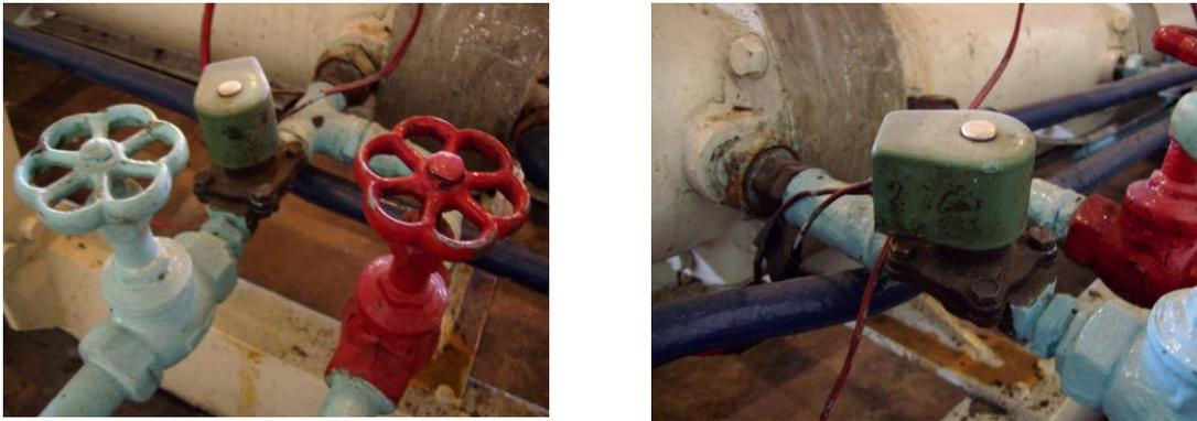
**FIG 7.6 ELECTROVÁLVULA MARCA ALCON MOD AC-236**
