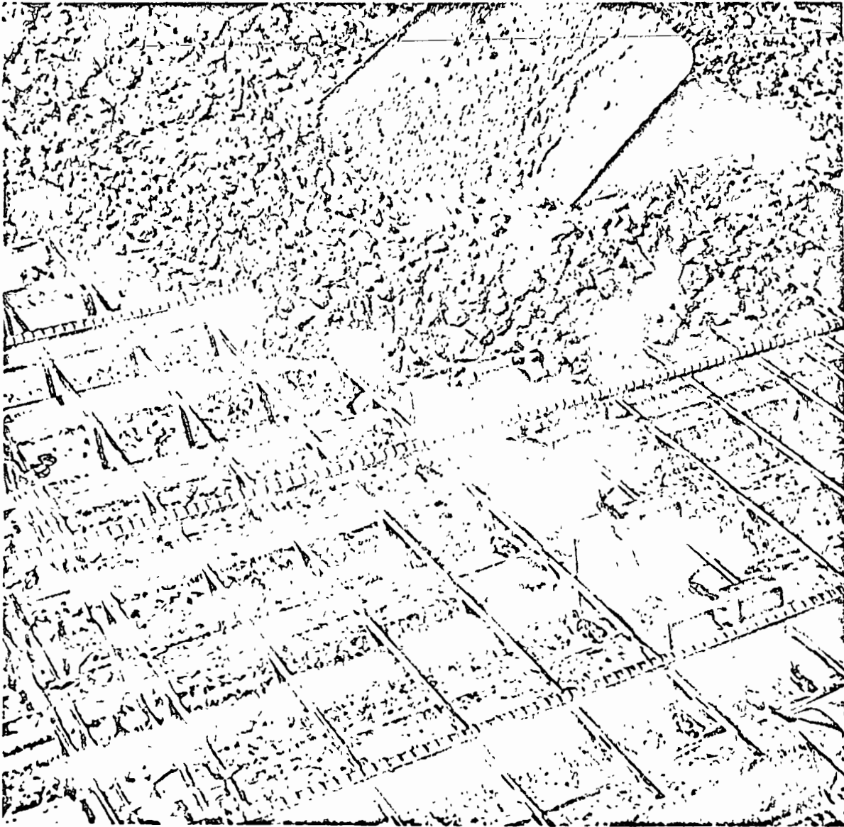
Application of one type of proprietary shear connector for composite construction, providing equivalent strength with less steel tonnage. Connectors welded to beams makes concrete slab integral with supporting member.
