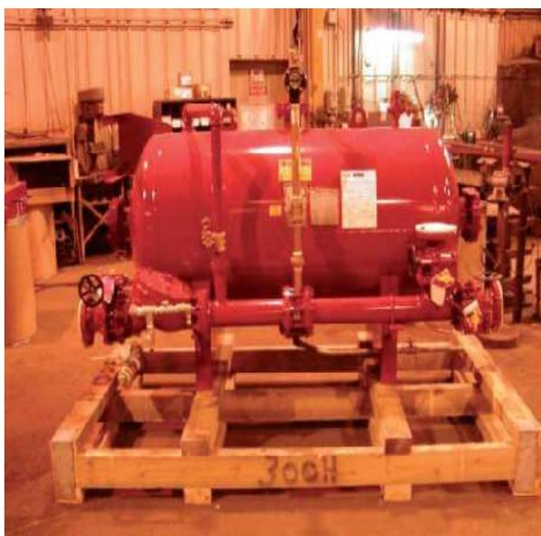
**Figura 2.7 SISTEMA FIJO DE ESPUMA.**
