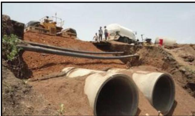
**Figura 2.2.3** Alcantarilla tubular de concreto
