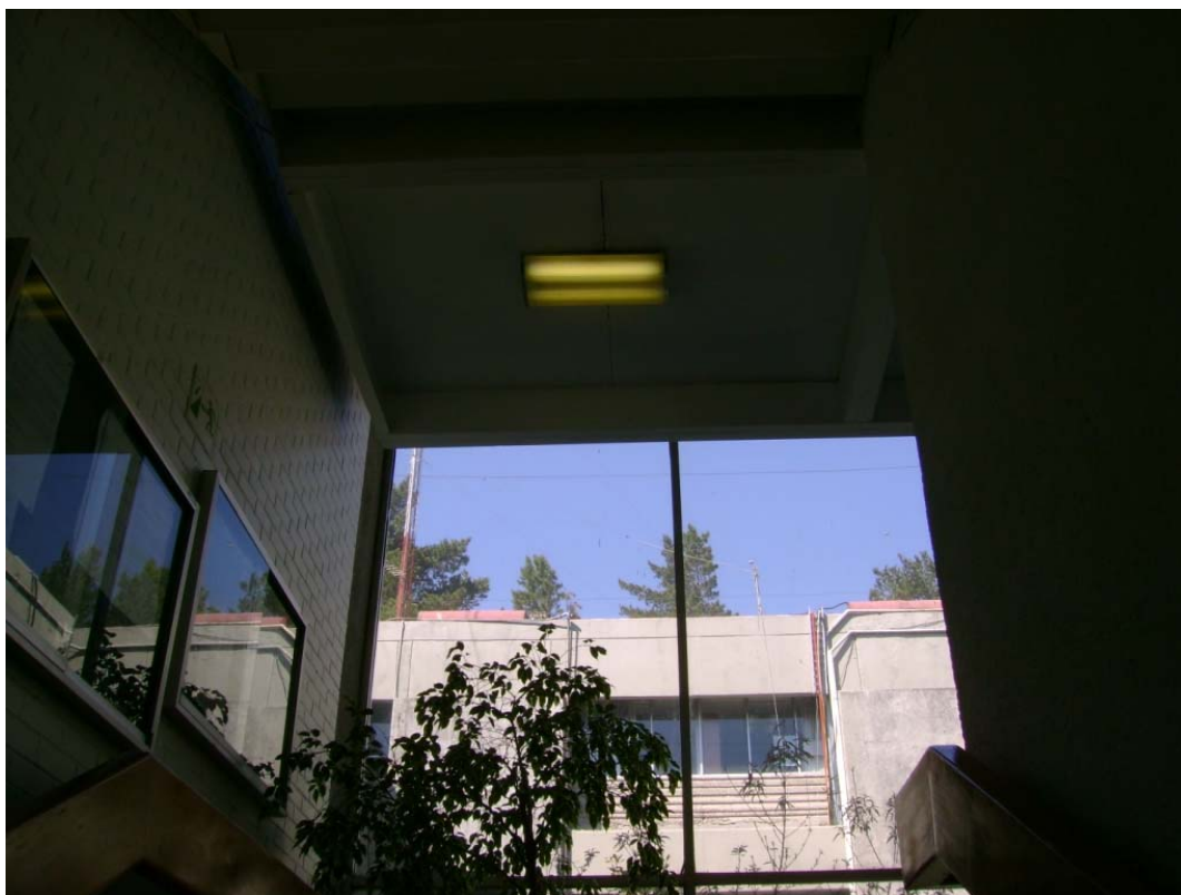
Escaleras PB-1N (10:44hrs)
