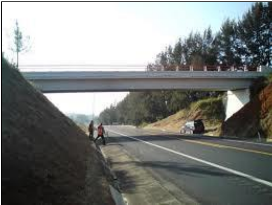
Figura 6. Paso Inferior Vehicular (PIV).
