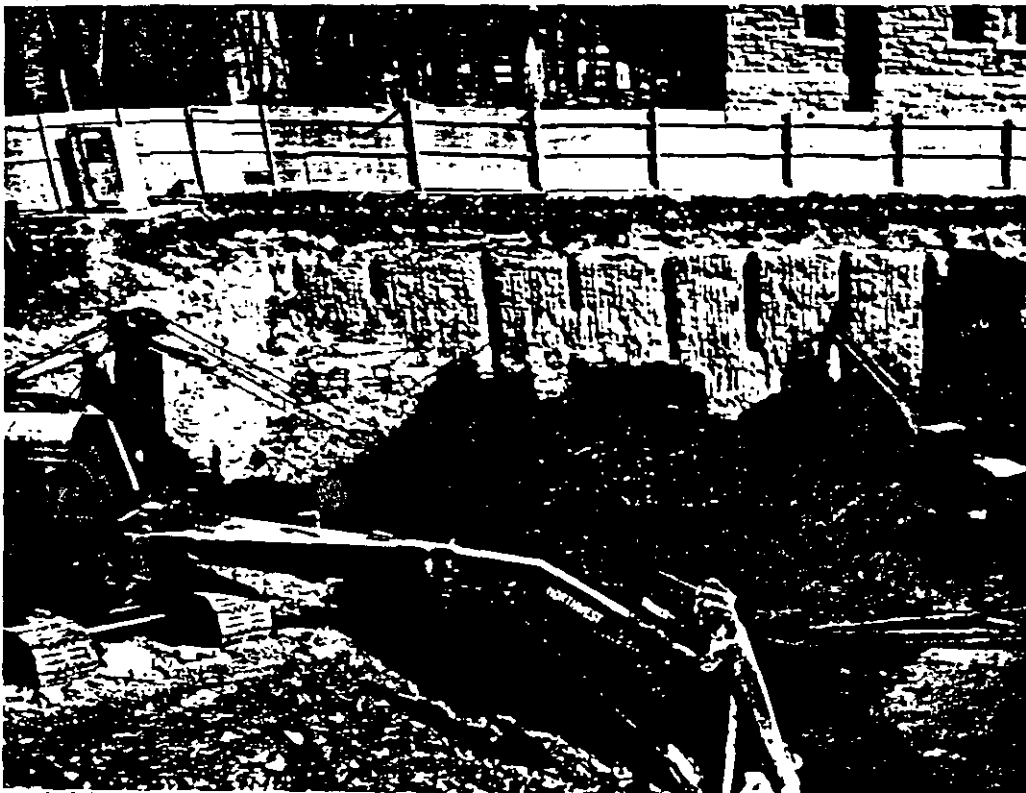
CUSHION BLAST RESULTS USING LARGE DIAMETER CUSHION HOLES AND SMALL DIAMETER GUIDE HOLES
